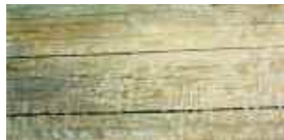
Felted wood after power washing.
